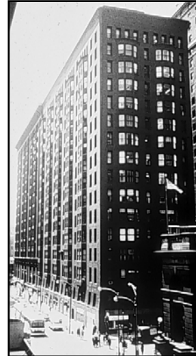
Monadnock Building, Chicago, 1889 URM 16 stories LB Unreinforced – 6 ft thick a base
