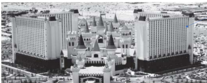
The four towers of the 28 story Excalibur Hotel Las Vegas – Load bearing masonry – ncma.org
