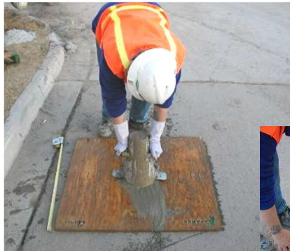
Self-consolidating grout Slump Flow
